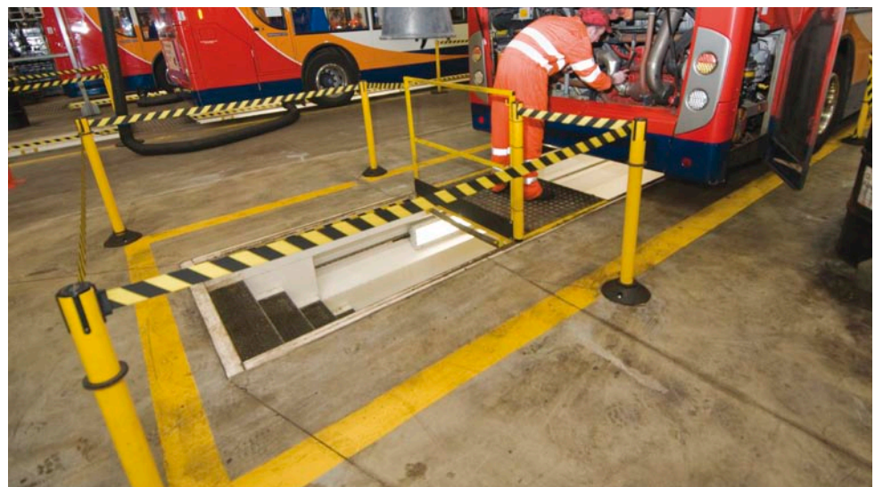
Figure 8 Extendible barriers warn workers about the open pit area
